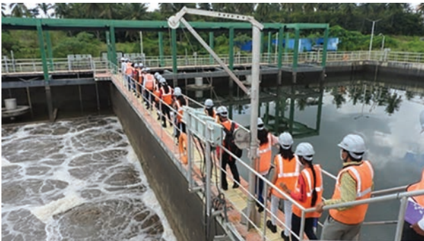
Wastewater Treatment Plant- Technician field visit – Doddabele STP
