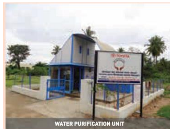
Figure 17: A photograph of one of the water purification units built as part of Toyota's CSR
